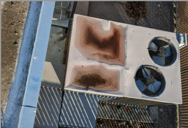
2 REPAIR DAMAGED SHEET METAL ON CONDENSING UNIT
