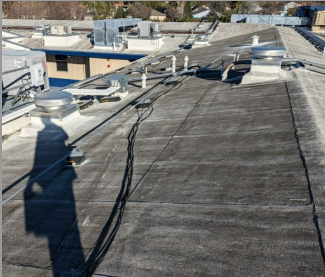
1 REMOVE DEBRIS (CONFIRM OLD COAXIAL CABLING IS UNUSED)
